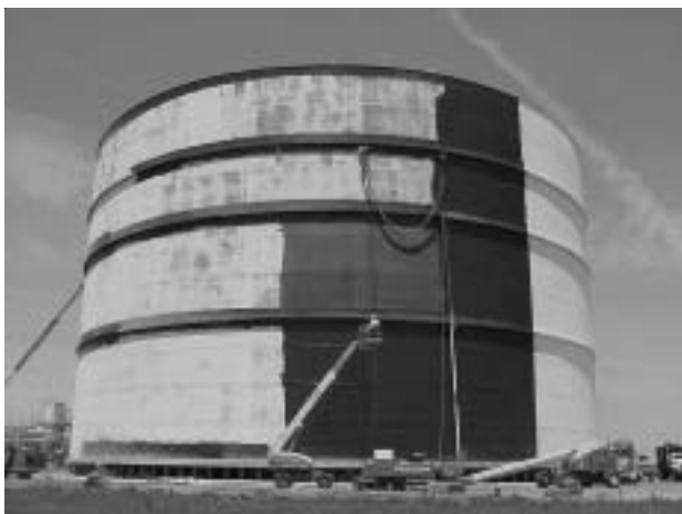
The SRT-10 Crawler beginning removal on a new section of tank.
