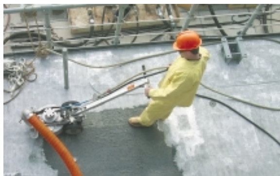
Coating Removal/Surface Preparation A lightweight SPIN JET® — an NLB exclusive — quickly removes coatings from floors, decks or grates.
