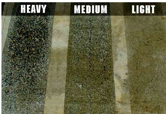
Various levels of concrete scarification
