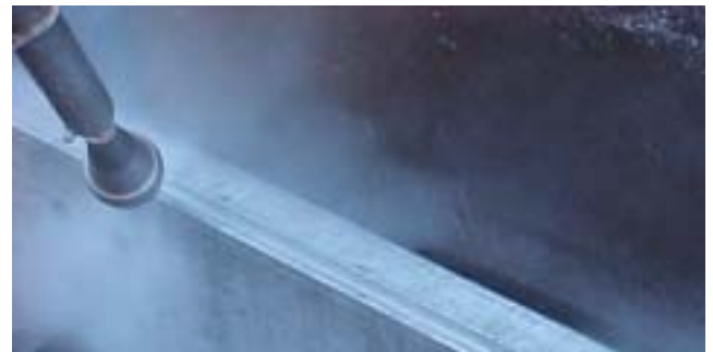
An NLB8400A-2 rotating lance cleaning out the concrete using ultra-high pressure water.
