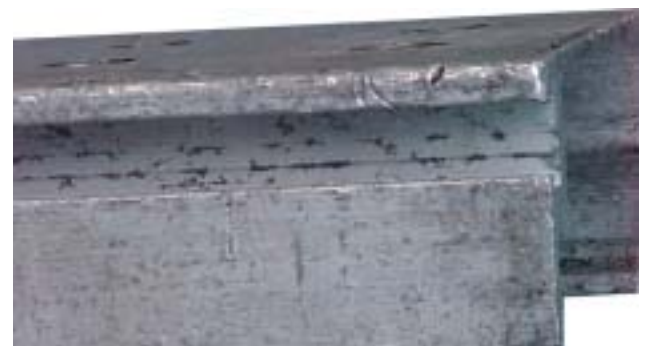
The "keyway" on the piece of staging with all concrete residue removed.
