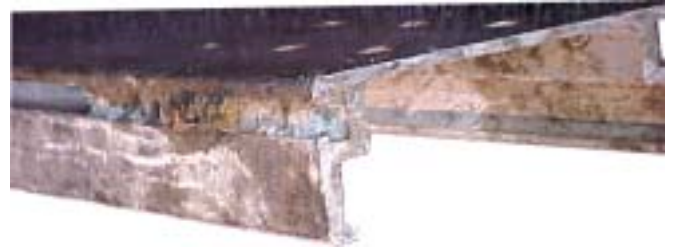
The "keyway" on a piece of staging filled with concrete.
