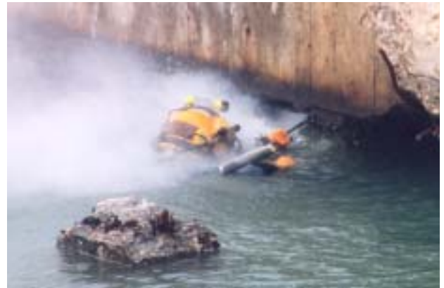
A diver working at low tide performs clean-up after a beam has been removed. One of the columns that was reused can be seen in the foreground.
