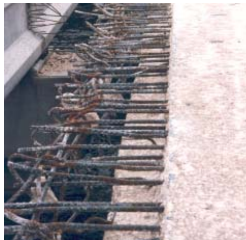
The NLB Concrete Buster efficiently separates the bridge rail from the bridge deck.
