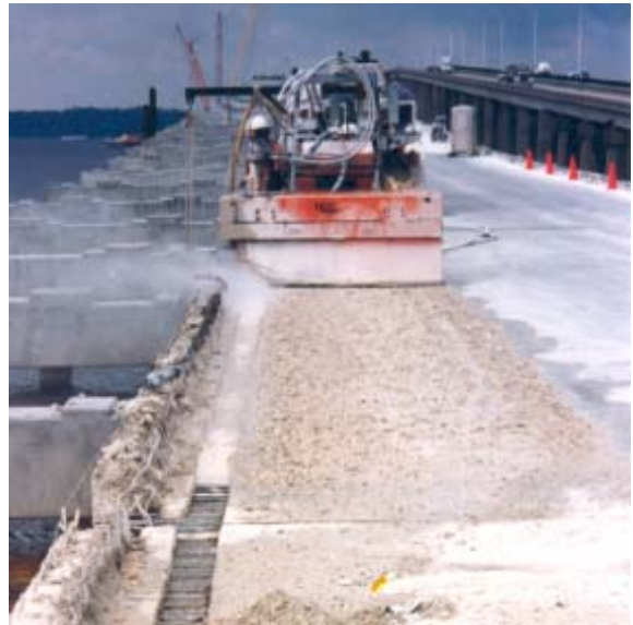
The NLB Concrete Buster efficiently separates the bridge rail from the bridge deck.
