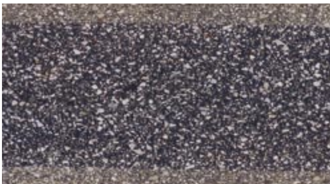
Water jetting completely removes stripes, without damaging the underlying pavement, better than any other method.
