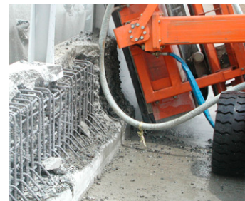
Concrete Buster 5500 for vertical hydrodemolition
