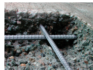
Hydrodemolition blasts away bad concrete, yet leaves rebar undamaged
