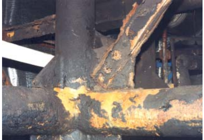
Section of piping before application of high-pressure water.
