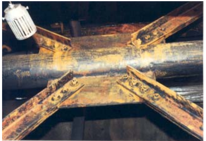
Section of piping after cleaning with 20,000 psi (1400 bar) high-pressure water.
