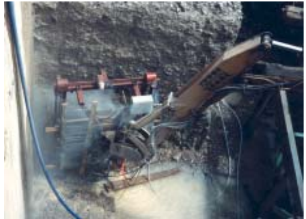
Unsound concrete is effortlessly removed from the vertical dam surface.
