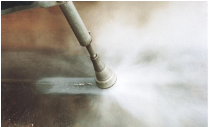
Water jetting is ideal for preparing ships, tanks and other large surfaces.
