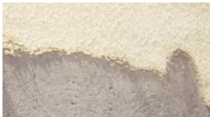
You can prepare concrete surfaces (shown here) as easily as metal.
